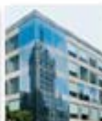
ATHENS, BUILDING B
